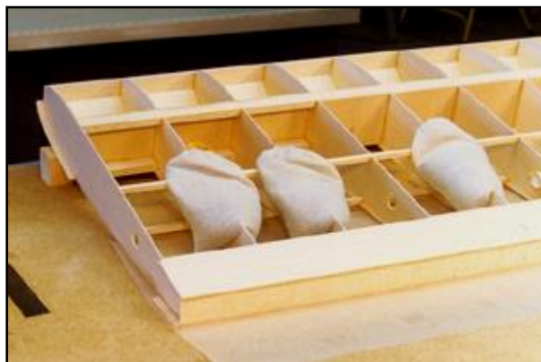
Wing Panel, Upside Down - The idea here is to position the top TE sheeting flat against the table. This requires a support at the front; I used a piece of lumber that was lying around. Worked well! You can see the TE sheeting overhangs at the rear. It will be trimmed later.
